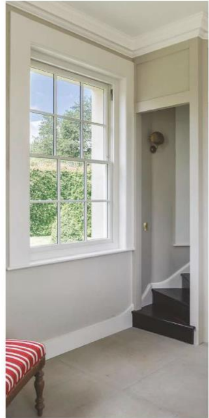
Fig 4: The stairs, with their curved skirting board, are ingeniously contrived against three internal sides of the octagonal plan
