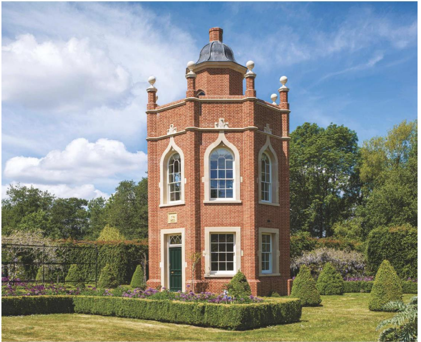
Fig 8: The folly is the centrepiece of the walled garden. The window surrounds, string course and finials are of reconstituted stone
